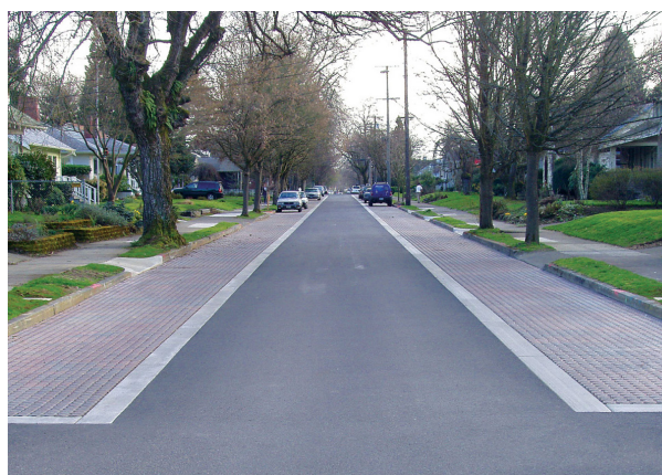
This street has a mix of impervious asphalt and pervious pavers, directing runoff to the parking lane where it can infiltrate the ground.
