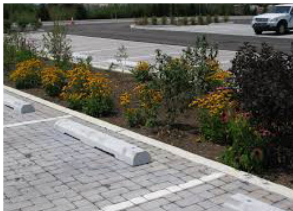
The parking lot is multi-functional, providing not only parking but filtering and managing stormwater runoff.
